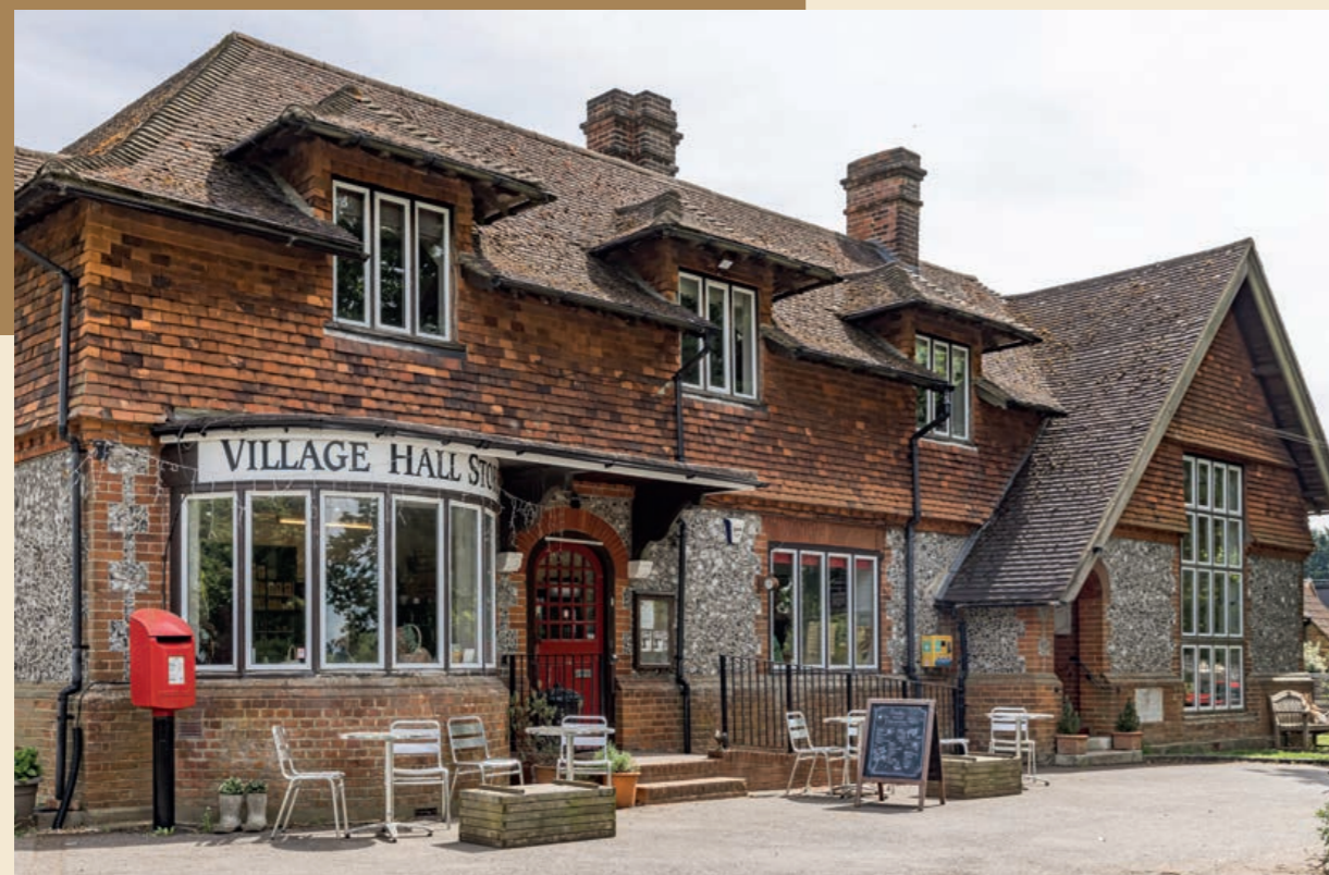
HEADLEY VILLAGE STORES & TEA ROOM
